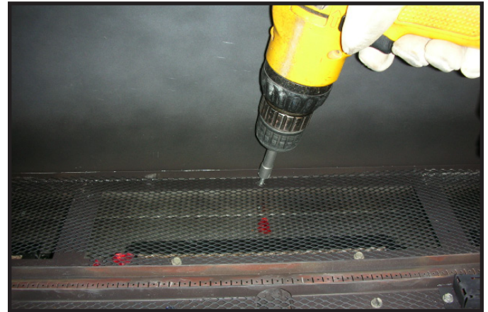
Figure 5. Removing Screws from Basepan.
